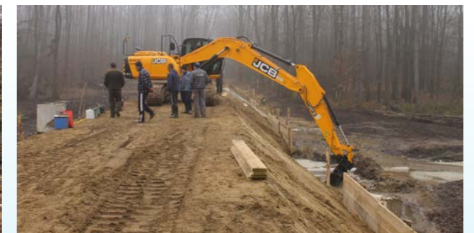
The new dam is under construction
